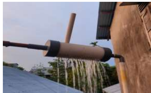
Pic 1. Aeration unit
